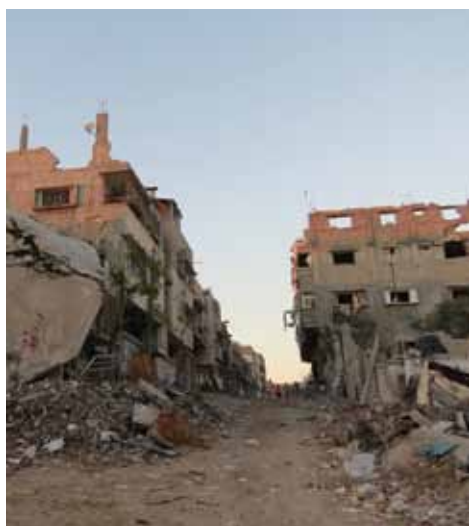
Destruction in Shuja'iya. Photo by HPH, 9 Sep 2014
