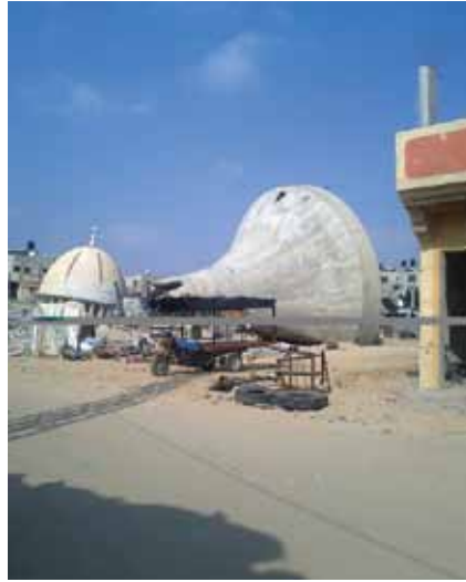
Destroyed water tower and mosque, Khuza'a. Photo by AV, 12 Nov 2014
