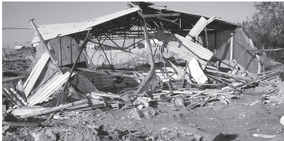
Figure 10: A destroyed agricultural storage building in Al Fukhari in the Gaza Strip. 135
